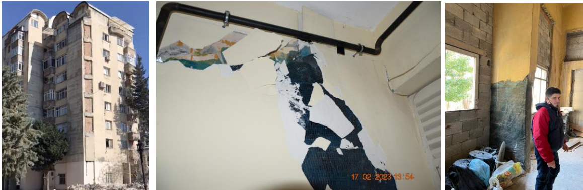
Figure 5.10. Performance of the strengthened building in Hatay
