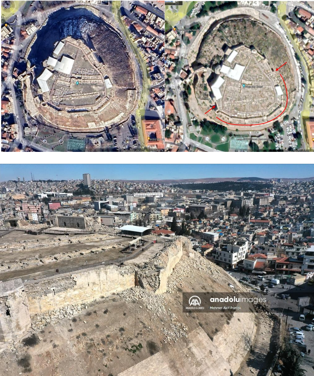
Figure 9.5 Gaziantep Castle before and after the earthquakes.
