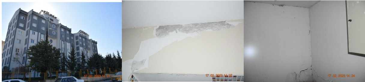
Figure 5.5. Performance of a tunnel form building
