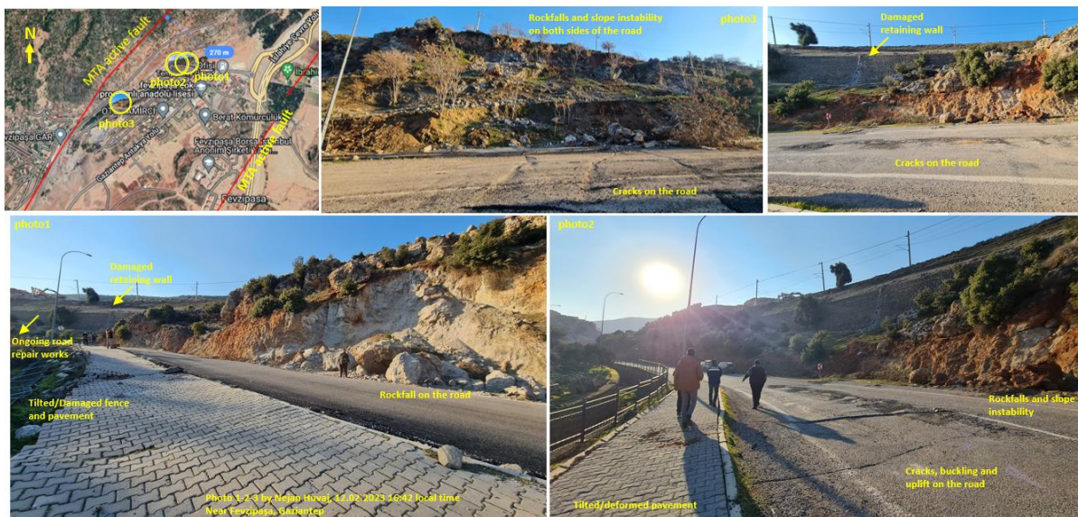
Figure 8.9. Landslides, rockfalls and surface cracks on the roads, near Fevzipaşa, Gaziantep causing disruption in the service (Active fault data from Emre et al. (2013)).
