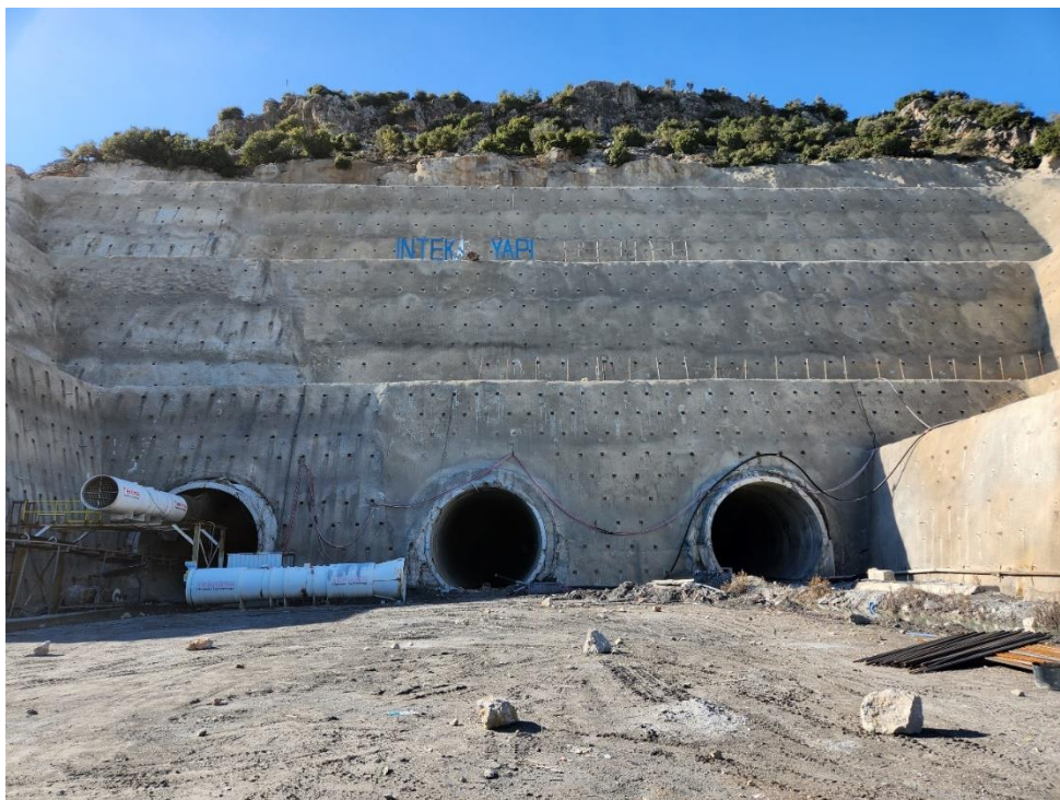
Figure 6.10. Nurdağı portal of Bahçe-Nurdağı railway tunnels
