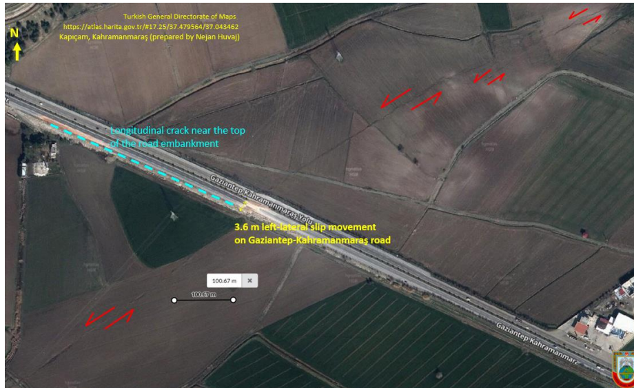
Figure 8.6. Surface rupture observations causing a 3.6 m offset on Gaziantep-Kahramanmaraş road, cracks on the asphalt road at several locations, road embankment instability and more than 250 m-long longitudinal cracks at the top of the road embankment as well as on the asphalt road, near Kıpıçam, Kahramanmaraş (Satellite images are provided by Turkish General Directorate of Maps via atlas.harita.gov.tr website)
