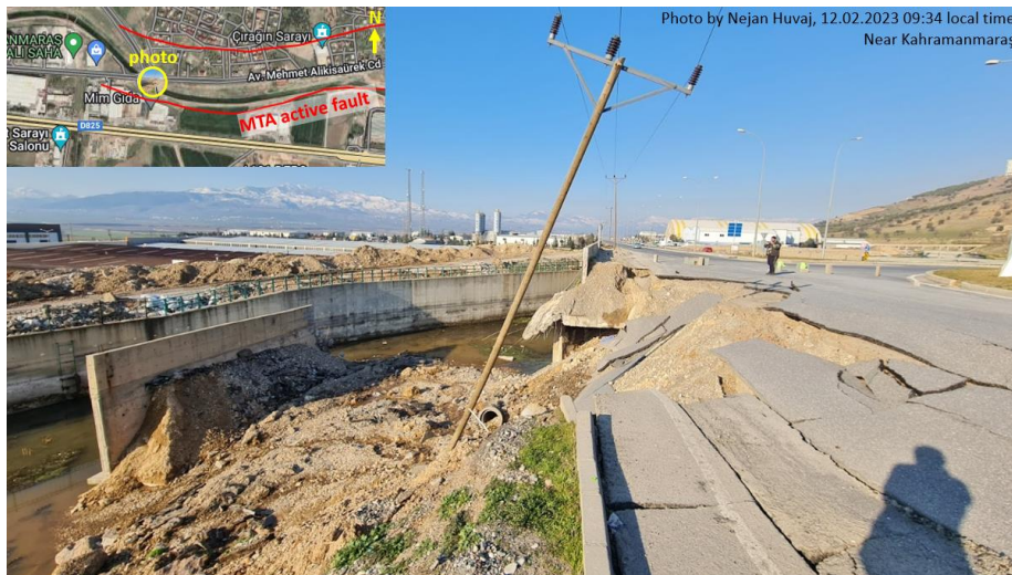
Figure 8.5. A landslide and crack/damages on the road next to a water canal, causing significant lateral displacement of a concrete retaining wall (pushed towards the water canal), a tilt on an electric pole, in southern part of the city of Kahramanmaraş (active fault data from Emre et al. (2013)).
