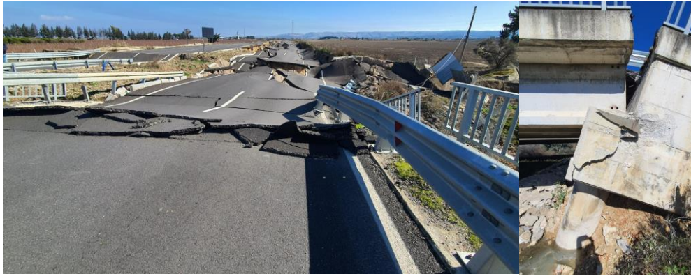
Figure 6.1. Abutment rotation due to seismic soil liquefaction induced foundation failure
