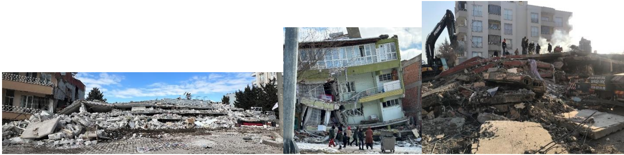
Figure 5.2. Building Collapse in Malatya
