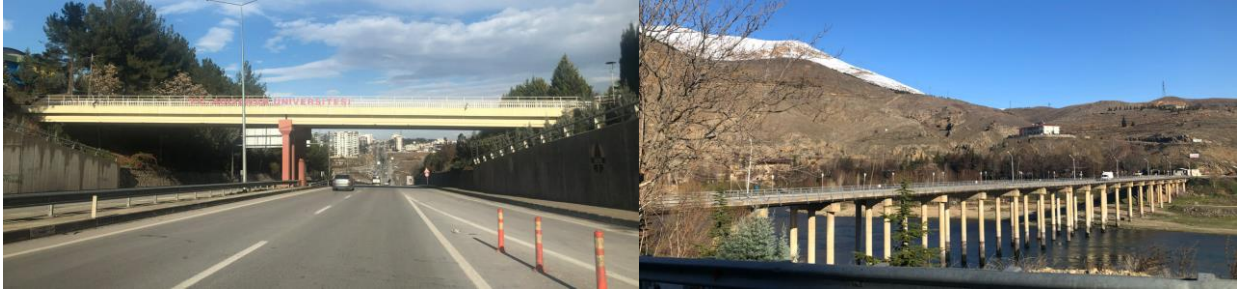
Figure 6.8. Bridge typical have no damage
