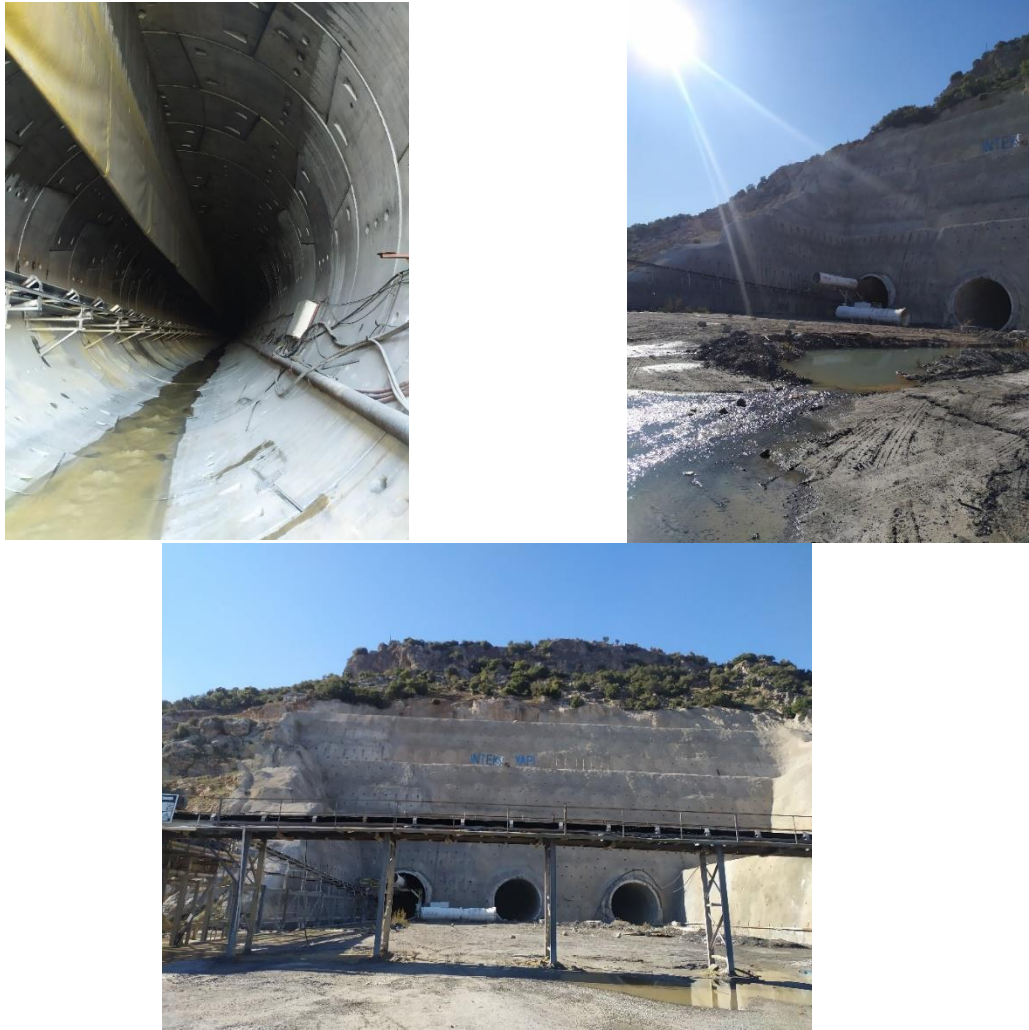
Figure 4.8. Bahçe-Nurdağı railway tunnels under construction in Nurdağı/ Gaziantep (37.16989°N, 36.70806°E)
