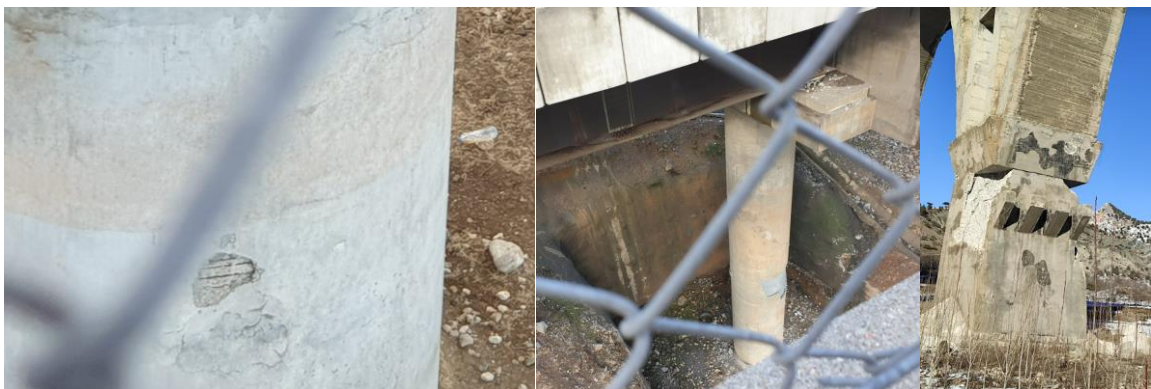
Figure 6.3. Concrete spalling
