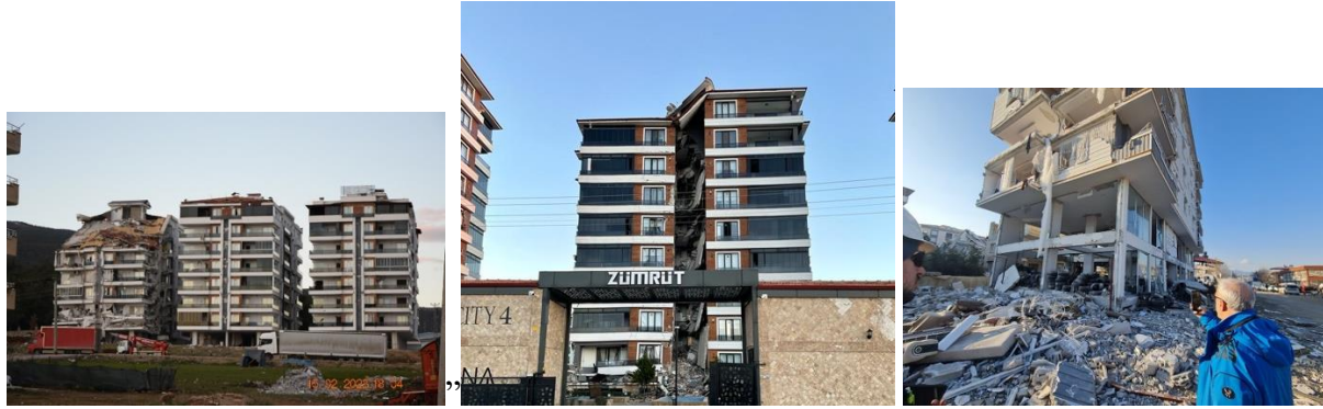
Figure 5.4. Heavily damaged new buildings in Adıyaman and İslahiye
